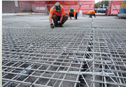
Glass Fibre Reinforced Polymer (GFRP)
